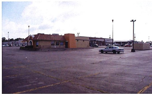
(left) Fast food parking lot; (right) Northern Lights parking lot - south end
